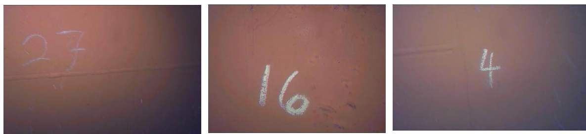
Fig.10a: Underwater inspection of VLCC tanker, 37 months after application with Hempaguard X7. No Hull cleanings, 70% activity, 27°C water temp, 12 knot operational speed
